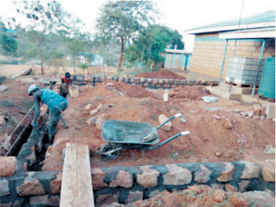
The foundations going in
