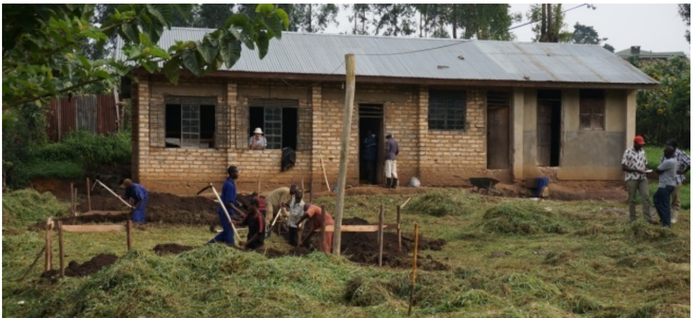
A 2014 Project Uganda project; behind is a dormitory built at a Girl's School , and in front foundations are being prepared for a new lavatory block.
