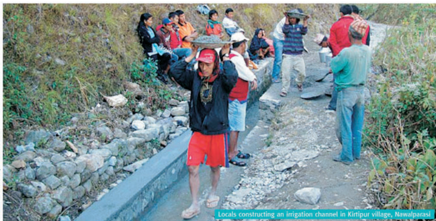
Locals constructing an irrigation channel in Kirtipur village, Nawalparasi
