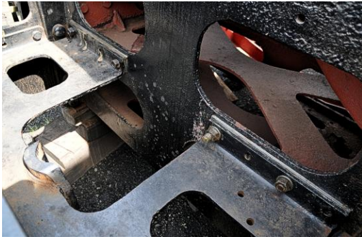
Front dragbox with spacers ready for riveting
