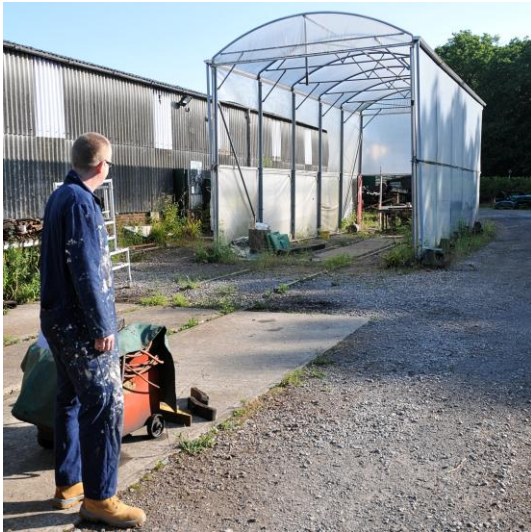
Ready to dismantle the poly-shed
